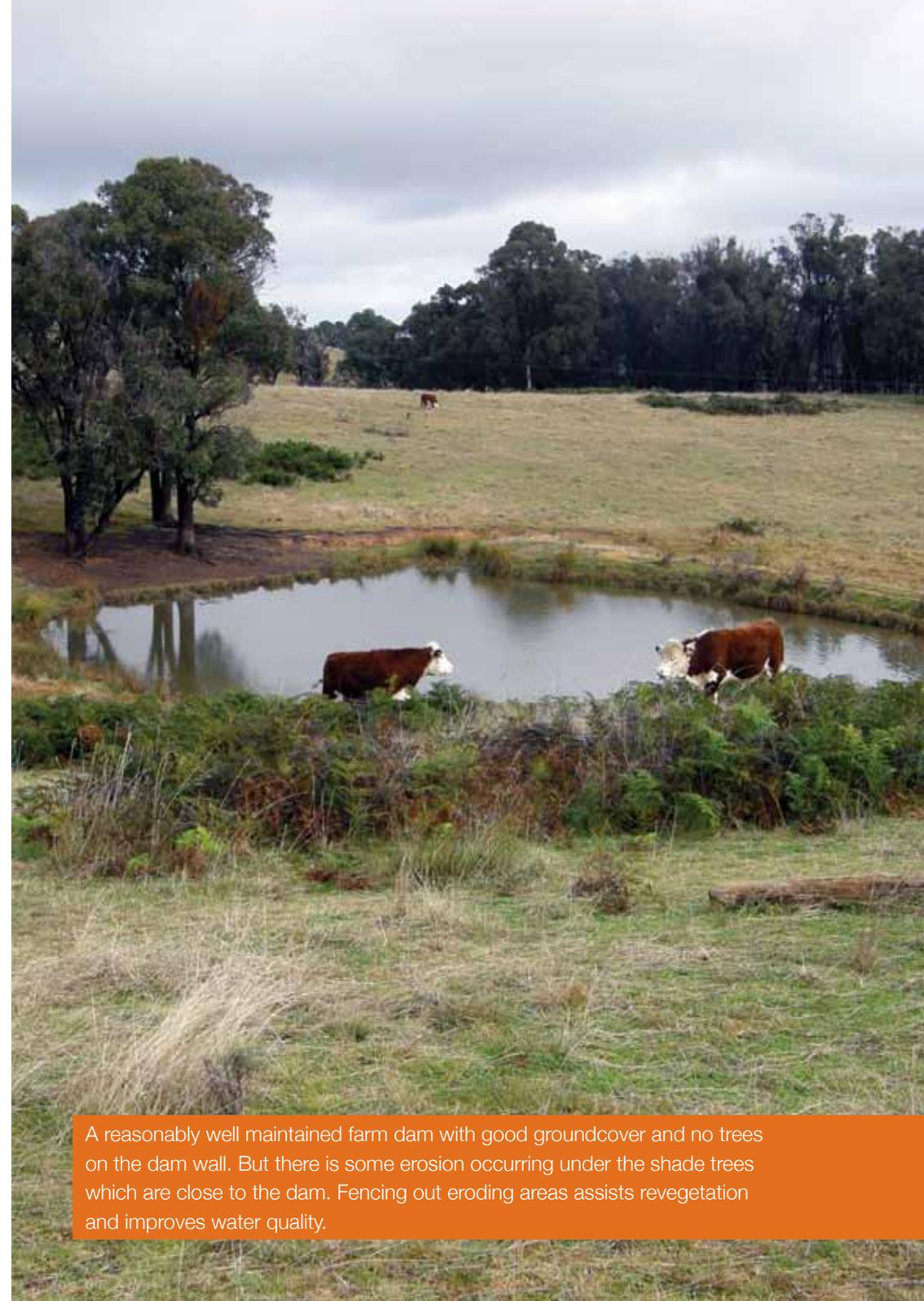
A reasonably well maintained farm dam with good groundcover and no trees on the dam wall. But there is some erosion occurring under the shade trees which are close to the dam. Fencing out eroding areas assists revegetation and improves water quality.
