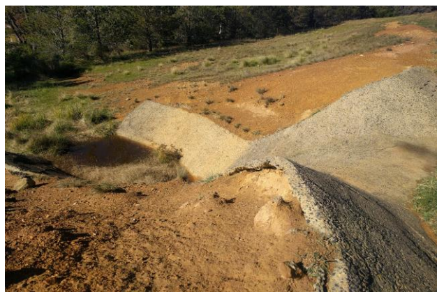
Fig 3: This unfenced flume has low surrounding groundcover which is under threat from further erosion
