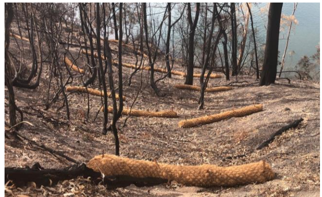
Fig 2: Coir logs installed to slow water and trap sediment.
