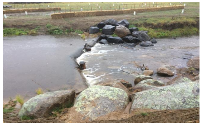
Fig 5: V-notch weir with rock, hay bales and jute mesh
