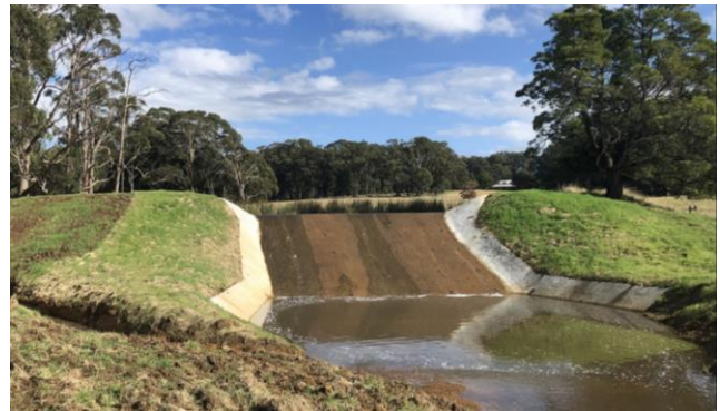
Fig 4: Concrete flume with long stilling pond.
