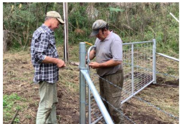
Figure 1. Installing new fencing.
