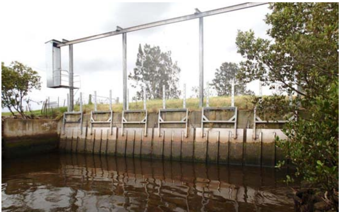
Figure D.2: P1 – Woodberry floodgates downstream
