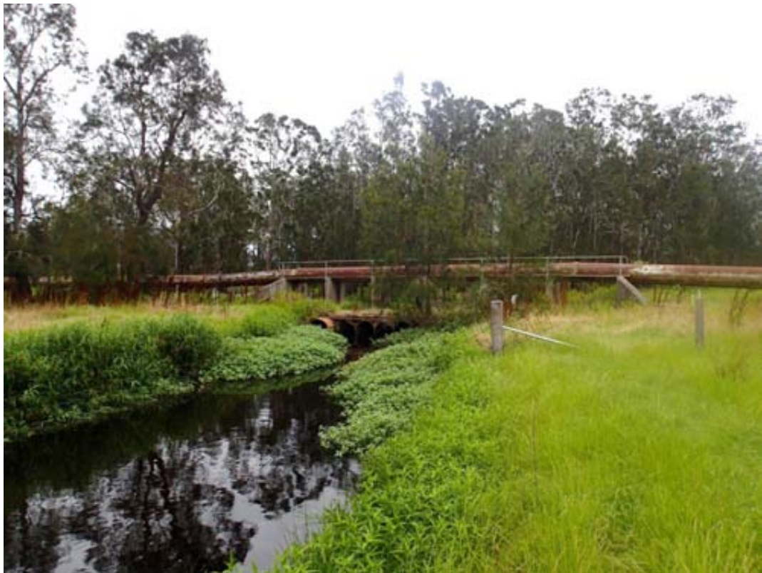
Figure D.6: P5 – HWC pipeline at Greenways Creek
