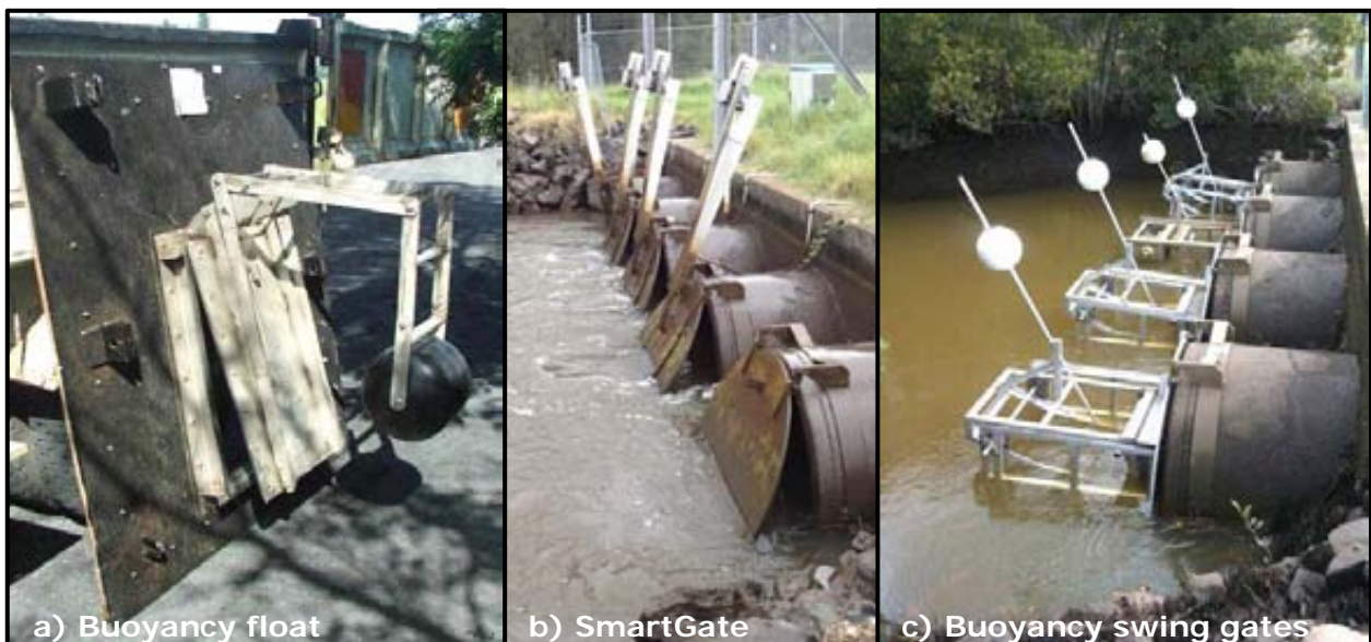
Figure 8.1: Different modified auto-tidal floodgate designs
