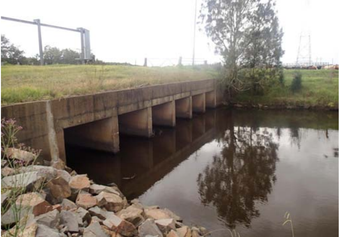
Figure D.3: P2 – Woodberry floodgates upstream
