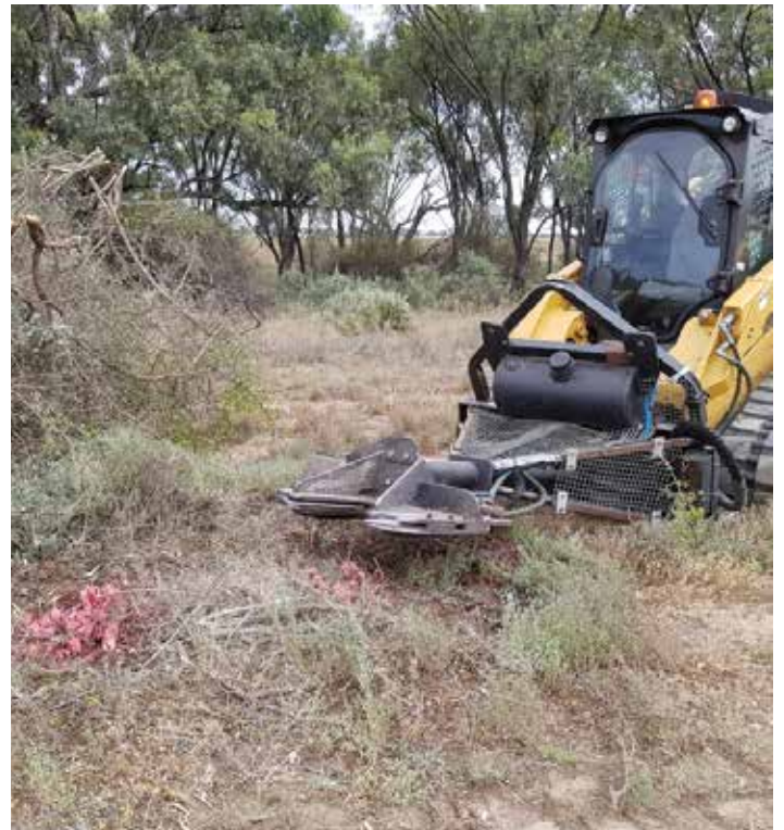
Boxthorn removal undertaken by Murray River Council.
