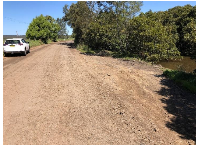
Figure 1. Mayfield Road prior to the works to seal it.
