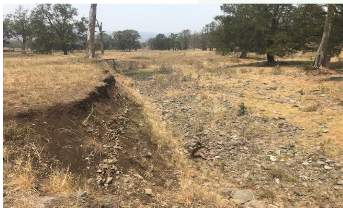
Big Jacks Creek prior to the rehabilitation project.
