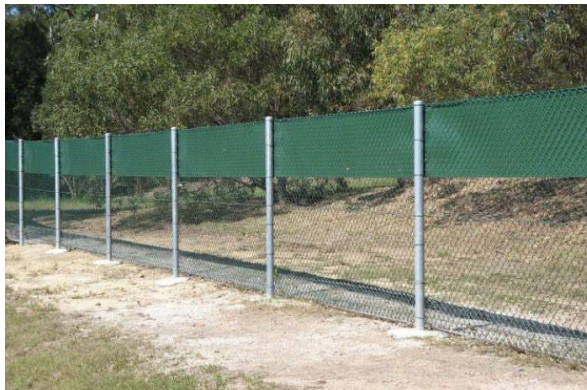
Figure A2: Koala exclusion fencing and fauna underpass with koala furniture. (Pictures from Koala Conservation Unit 2012)
