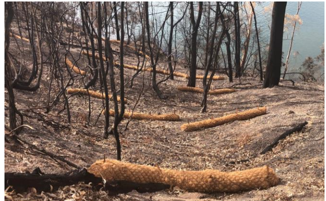
Figure 1: Coir logs and large woody debris pinned across a steep slope to slow water and trap debris and sediment.
