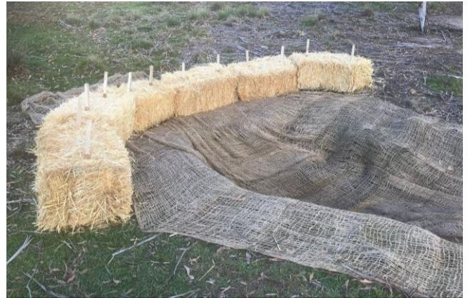
Figure 6: Jute mesh and straw bales pinned across this slope with hardwood stakes to slow water flow into head cut.
