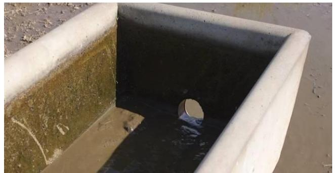
Figure 7: Empty the trough and clean regularly to remove sludge accumulation. Photo: South East Local Land Services
