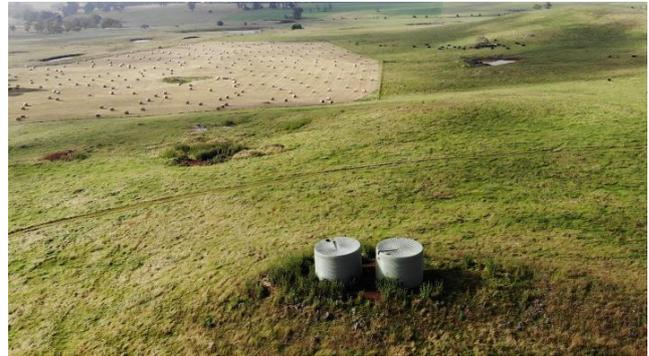
Figure 4: Tanks located on hill so that water can gravitate to troughs, this can eliminate the need for extra pumps
